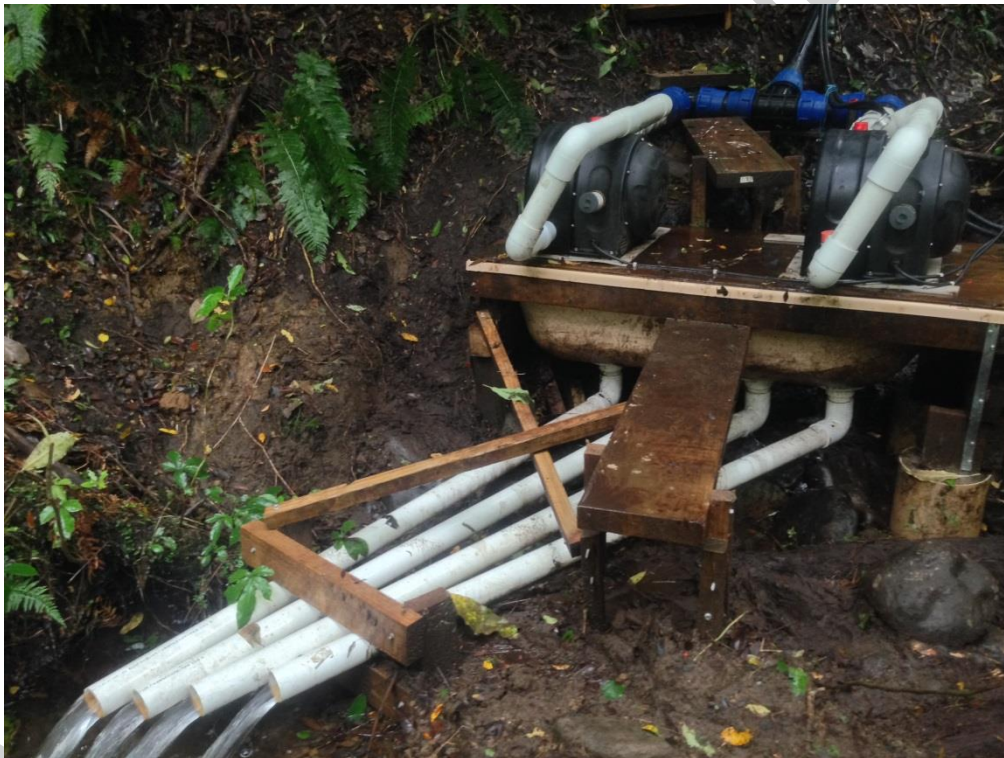
Close breakers and turn turbines on
