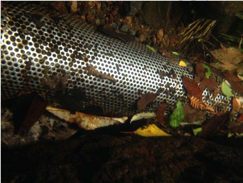
Intake after 1 day of operation – is it not an adequate solution
