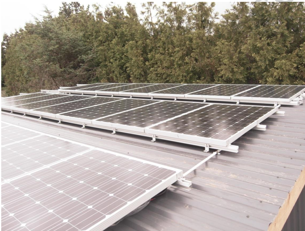
5.25 kW PV array was installed to allow the home to be built over the summer 21 x 250W panels in 7 strings of 3 (ELV)
