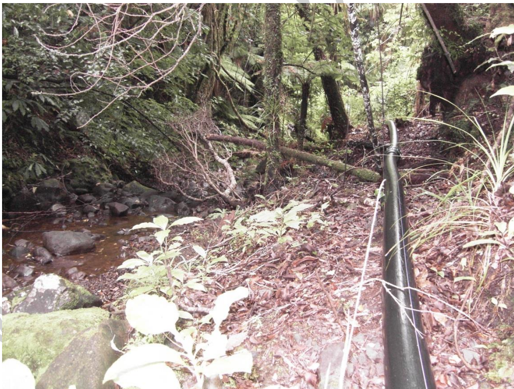
The pipe was laid by the owner, the terrain becomes very difficult in places and this resulted in about 15 high points that needed to be vented to prevent air locks.
