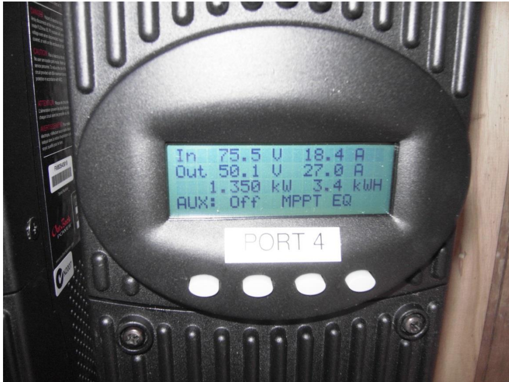
Output varied from 1340-1430 Watt, prior to sorting out intake issue. MPPTV 76VDC, PV trigger was set to 85 VDC
