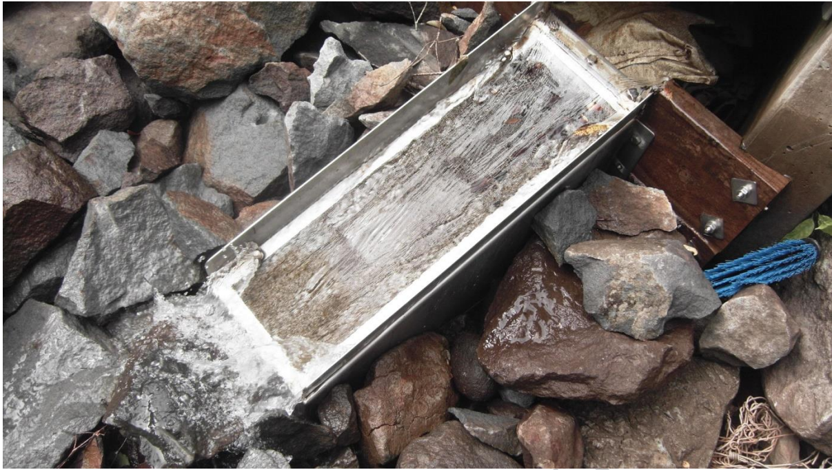
Upgraded inclined intake made from stainless steel. This is one of the most important parts to get correct, do not cut cost on the intake.
