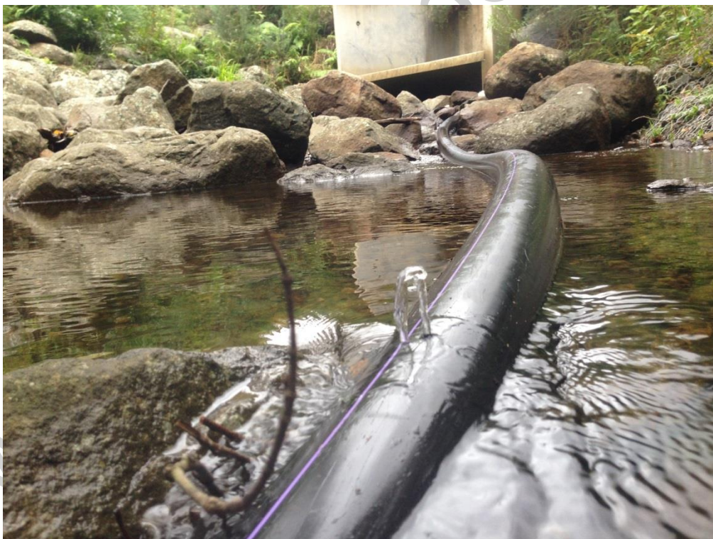
The pictures shows a 4mm hole drilled in the pipe, 15m down from the intake and about 800mm lower. There is very little pressure as can be seen from the low height of the water jet. An improved intake design will help. Always try and get a good fall on the initial 20 m of pipe if possible. In this example a partially blocked intake will result in negative pressure at this vent, which can draw air into the pipe line. The concrete structure in the picture is part of a road culvert (a convenient place to put the intake for access). It is not part of this hydro scheme.
