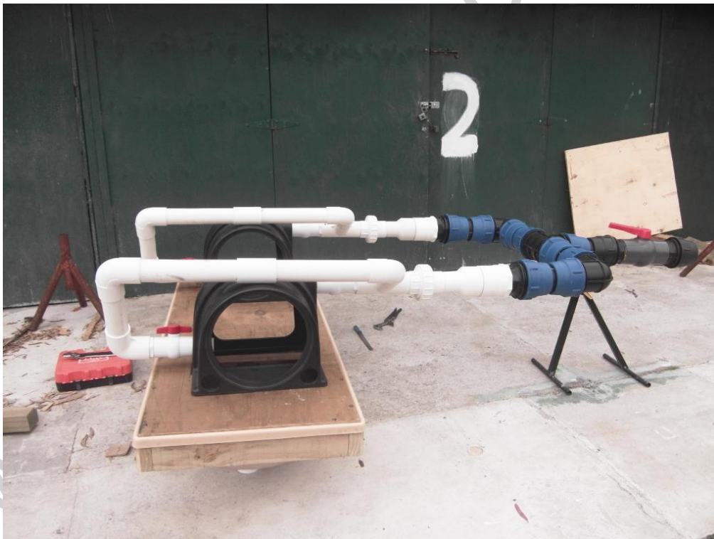
Mock-up of turbine and pipe manifold prior to carrying parts 800m into the bush. Do as much work as you can close to a workshop and not at the site. This will save time and keep costs down.
