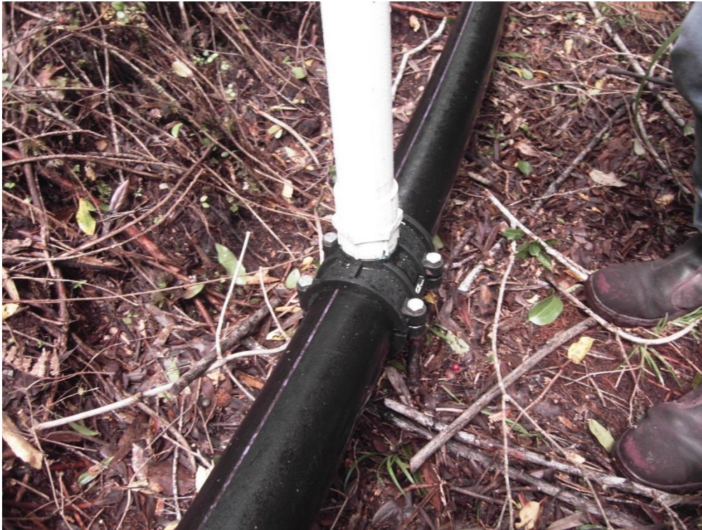
A large vent was fitted at the first high point to allow air to escape
