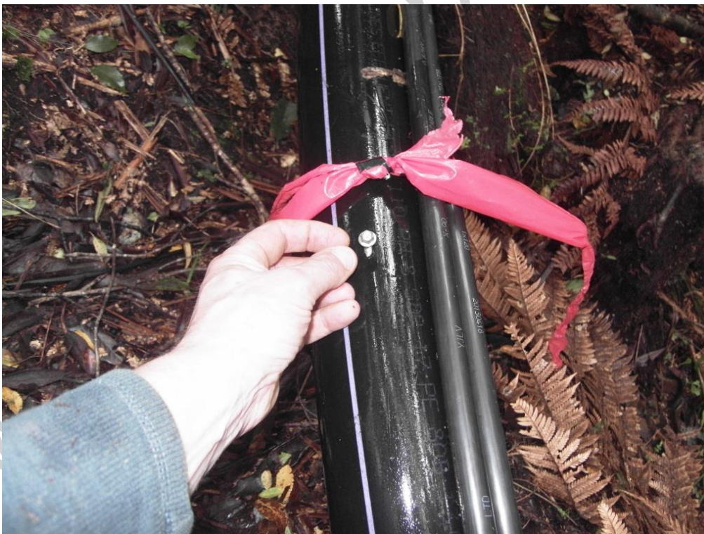
At the other 14 high points stainless screws were inserted and allowed to weep. This method purges air locks while only allowing a small amount of water to escape the pipeline. Note the red tape is used to mark these positions so they can be easily located in the future
