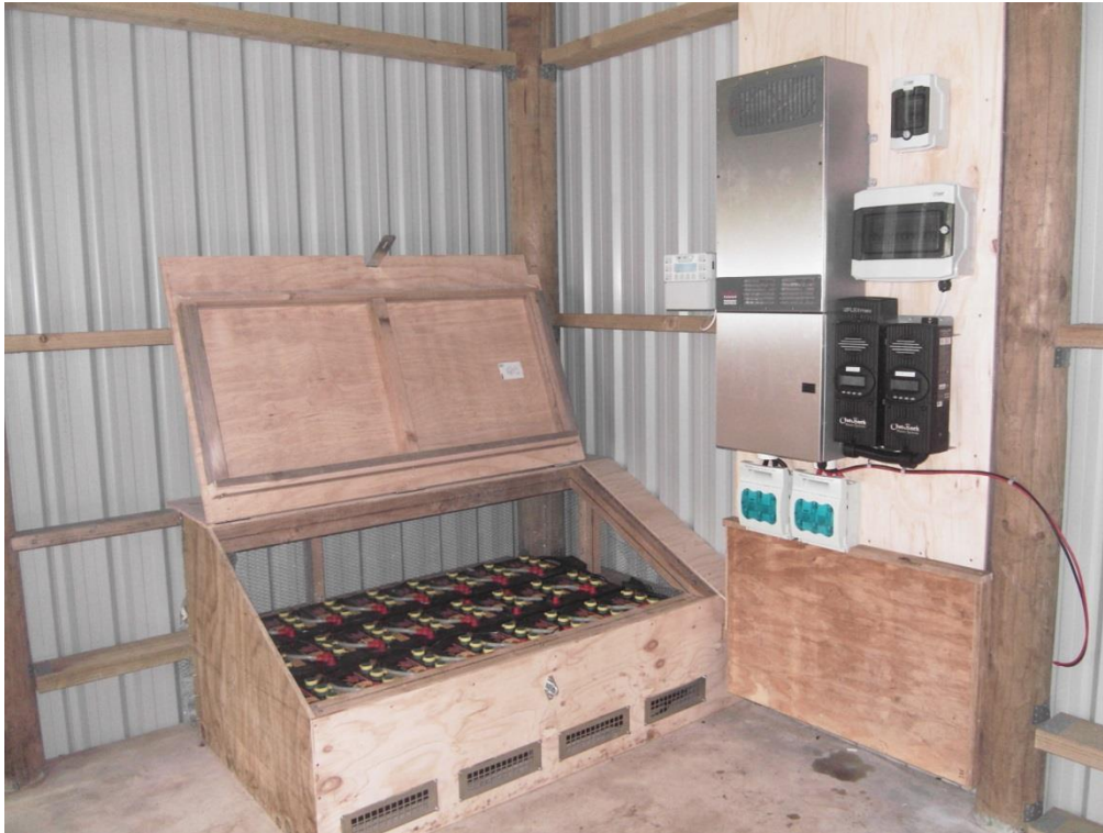
7kW Outback Radian system installed with FM60 ready for hydro input - once turbines installed
