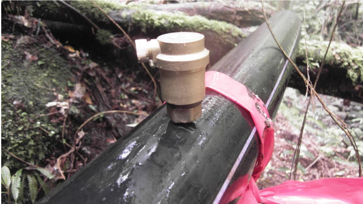
Upgrading temporary air release vents to automatic air release valves.
