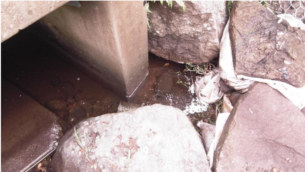
The client made a small temporary perforated tube intake. These are generally not suitable and will block quickly with leaves as shown. The client upgraded this is line with our advice in the installation manual.
